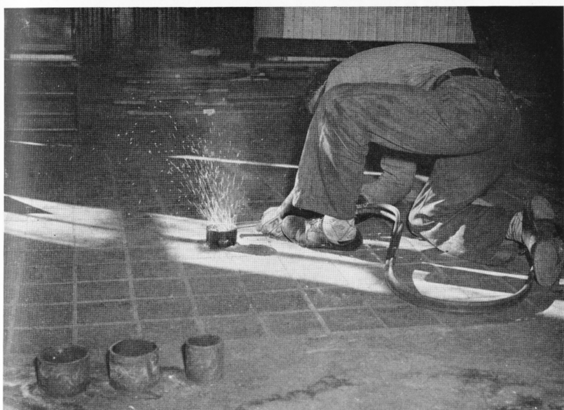
Ralph Orsini had the job of cutting jutting pipes flush with the floor in the game room. These pipes formerly carried water and heat. Here SERA members will be able to play pingpong, pool and card games. This room was on the right of the hall back of the stage, and was used for storeroom, scenery and dressing room at activities.
